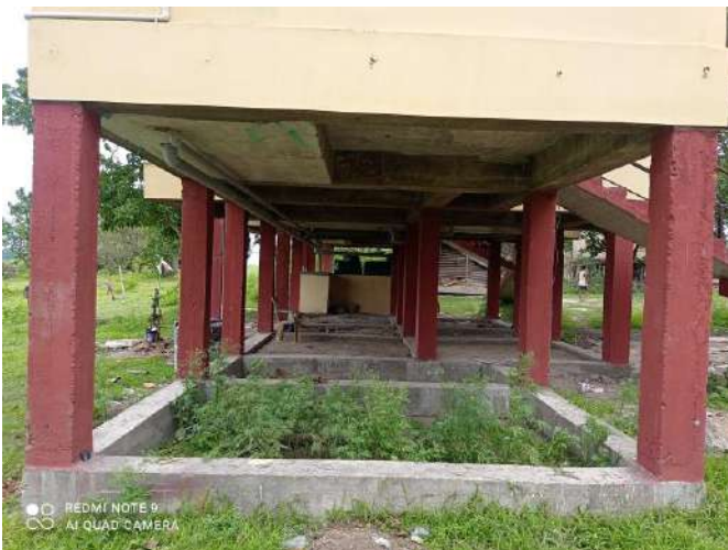
Concrete Columns to elevate the structure above the flood line
