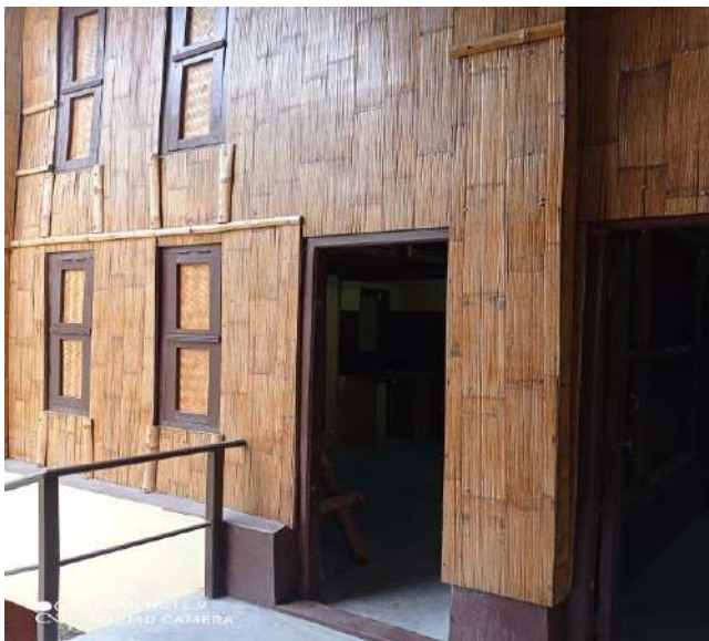
View of Bamboo boards on the exterior walls
