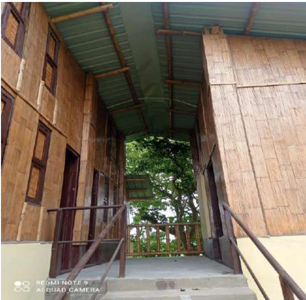
View of Passageway and Roofing
