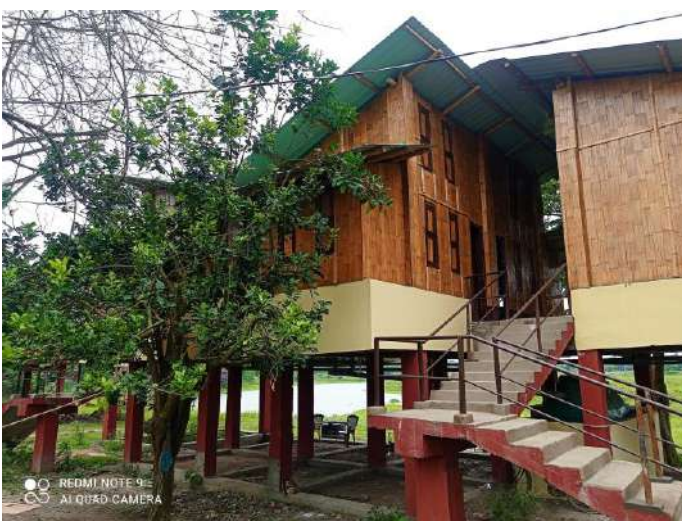
Roofing for ventilation and protection from Rain
