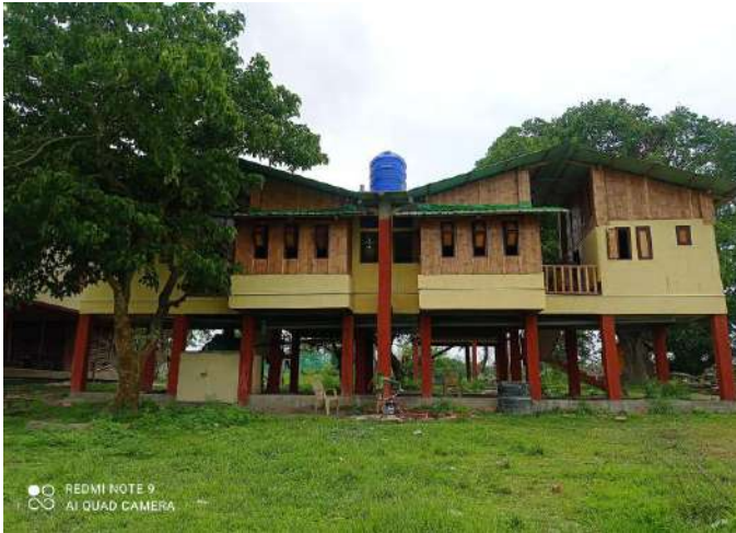
View of completed Barracks from access road
