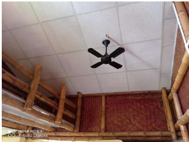
Roofing for insulation in each unit
